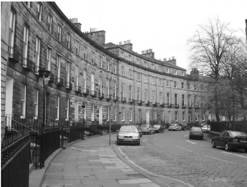
4.1. Edinburgh New Town achieved considerable architectural cohesion through the widespread choice of neo-palladian and neo-classical building styles.
