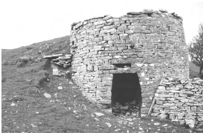
2.6. A field kiln near Ravenstonedale in Cumbria, which shows how kilns were, where possible, built into banks which facilitated the top loading of the kiln with limestone and fuel. Such kilns were usually intermittent in operation and were often associated with particular farms (by kind permission of Marilyn Palmer).
